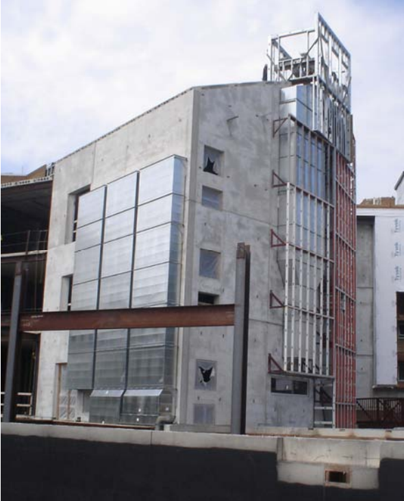
Figure 5: Pre-cast concrete structure with supply air ducts (left) and return air duct/stack (right), during rough framing. Source: (Author 2006)
