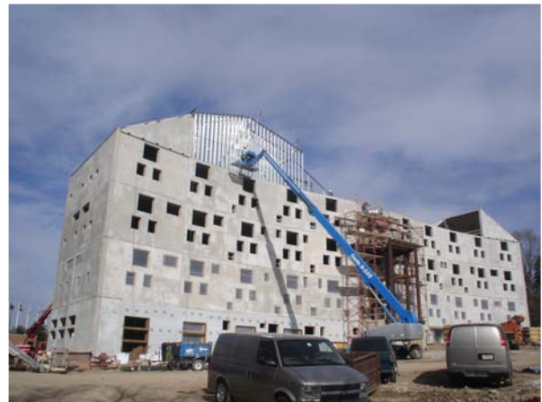
Figure 3: Pre-cast concrete structure. Source: (Author 2006)
