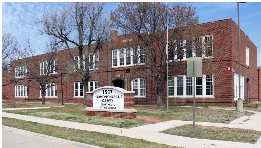
Figure 16. External view of Marcus Garvey Harmony Apartments as of today. Source: Authors.
